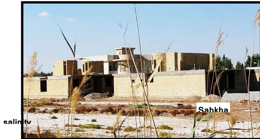
Figure (12) The salinity of agricultural soil and its extension towards the walls of the houses in the Al-Dahira region. Field study on 12/4/2022.
